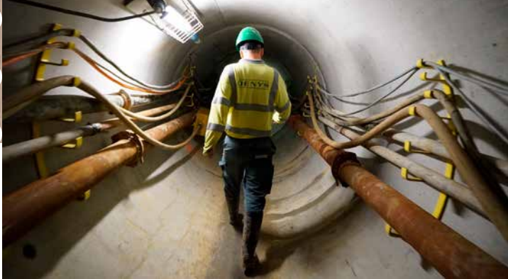
Two micro-tunnels were built for the pipeline to cross the Saône and Doubs Rivers.
