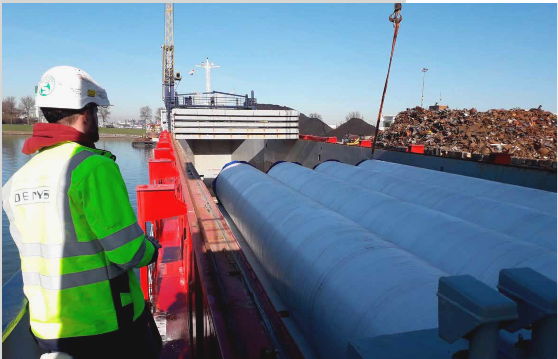
Three parallel 2.100 mm diameter pipes will be laid into the river bed using the off-bottom tow method.
