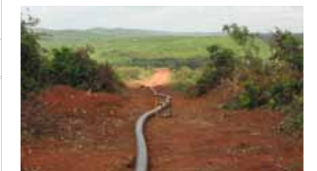
The dam captures no more than 5% of the water stream, leaving the river undisturbed.
