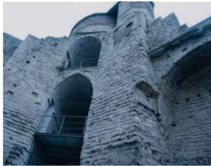
*We needed to build against the curtain wall an auxiliary construction, anchored more than six metres below the tower's foundations.*
