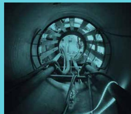
We used micro-tunnelling to cross the high-speed rail and the A16 highway.
