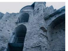
We needed to build against the curtain wall an auxiliary construction, anchored more than six metres below the tower's foundations.
